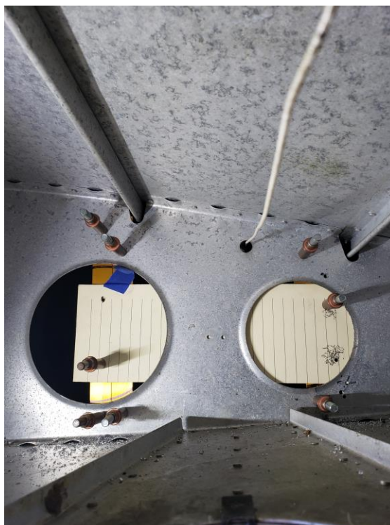
FIGURE 4-4 RIB STIFFENERS FIT
