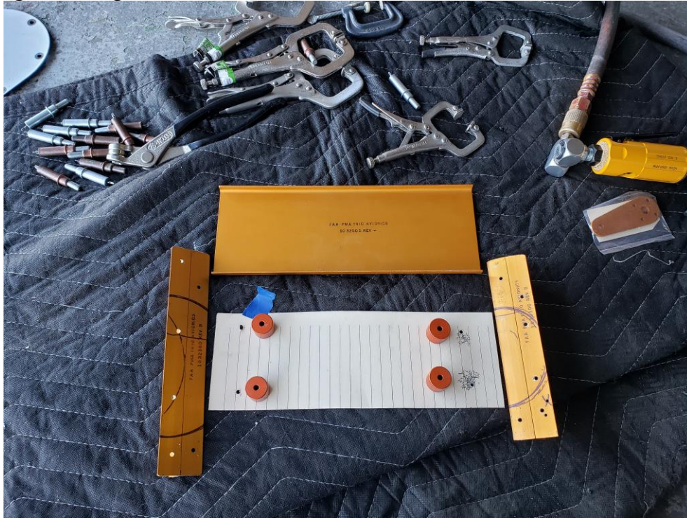
FIGURE 4-5 FINAL FIT CHECK
